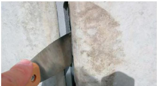
Due to security reasons the tape should be recessed in the joint by at least 2 mm from any radius or edge. The tape must not line up precisely with the edges of the joints!
